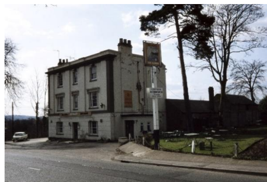
A later view of the hotel showing the roadside pub sign and adjacent garden seating, c.1980. Image: P2015.2638
