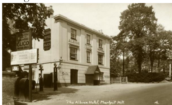
The Albion Hotel, Albion Garage and Marlpit Hill Service Station, after 1950. Image: P2014.2295
