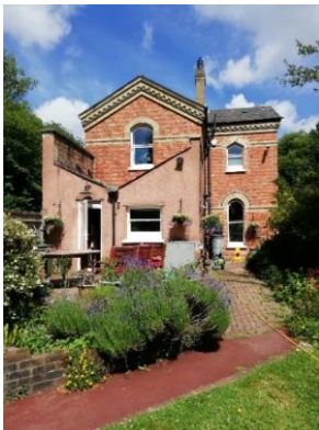
South aspect of the Station House showing exposed valley roof and the new window (bottom right) added to afford a view of the garden. Image: © Joan Varley, 2022
