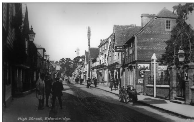
Edenbridge High Street looking north with entrance to Oddfellows Hall on right, c.1920-1930.
